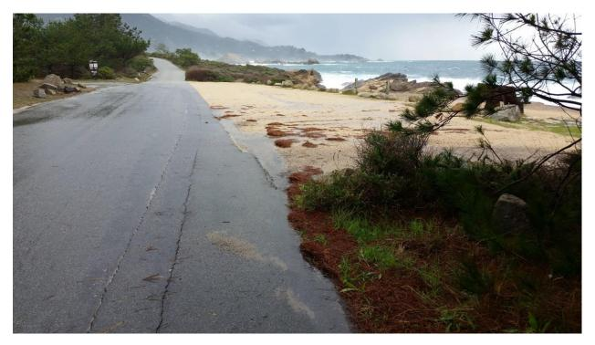
Figure 29: Water running down the road into the Piney Woods beach parking area. This increases the rate of bluff erosion by directing runoff onto the devegetated parking lot and bluff.
