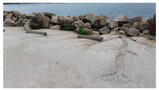
Figure 34: Erosion of the Whalers Point parking area into the ASBS.
