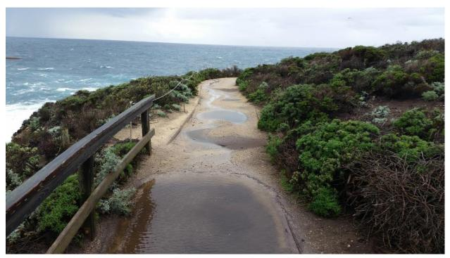
Figure 27: Ponding and running water on Sand Hill Cove Trial. Lack of water control features leads to sediment transport and trail degradation.
